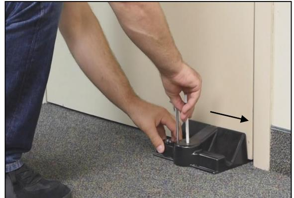
Fig. 1 – Using device to mark Floor Anchor Hole™
