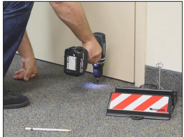
Fig. 2 – Hole Saw in Reverse on Carpet
